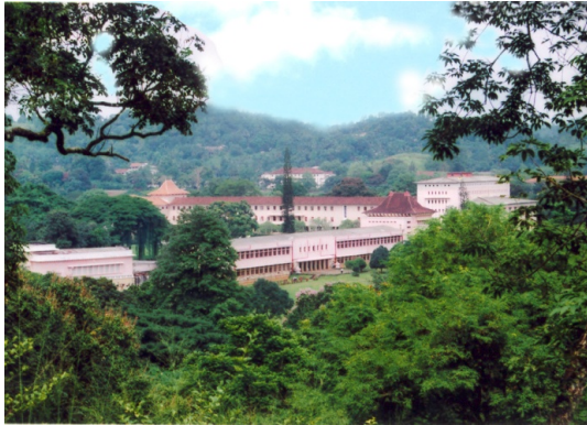
Aerial View of University of Peradeniya
